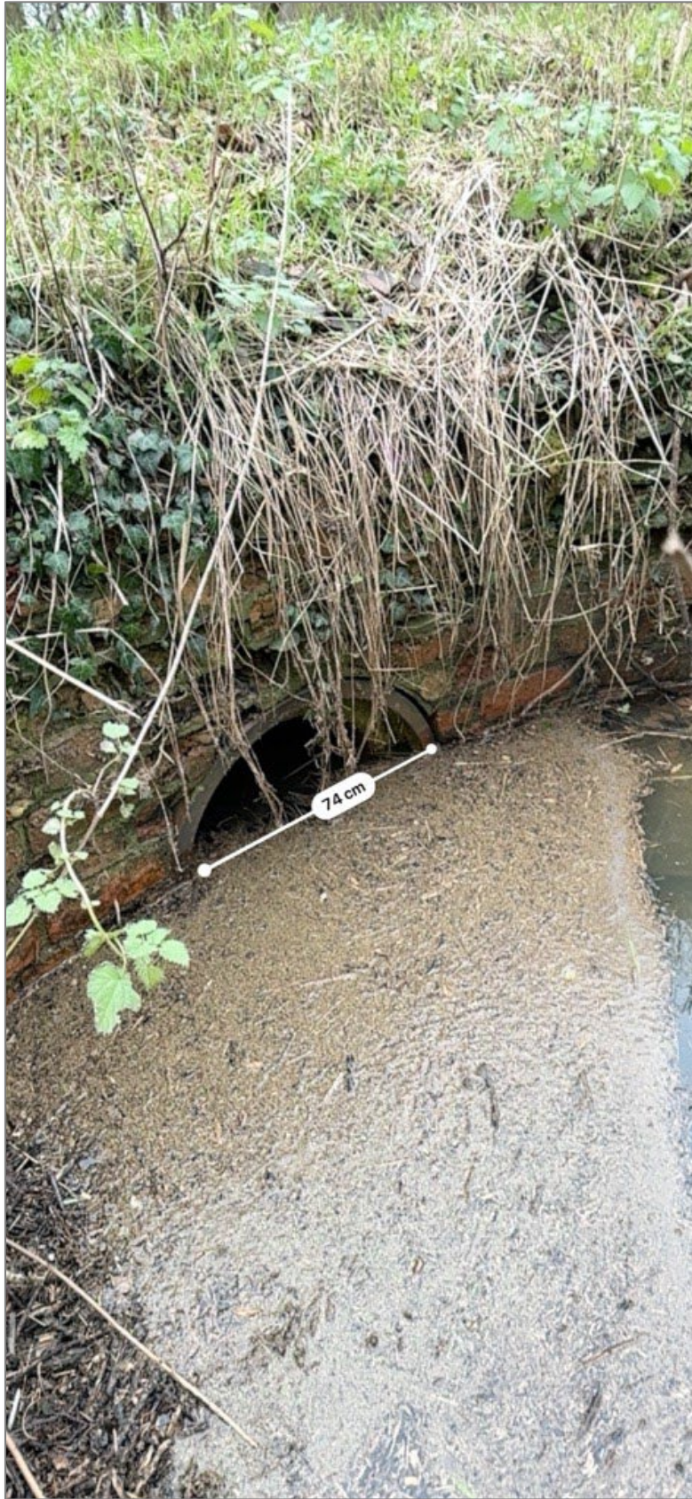
Figure 11: Upstream face of the Station Road culvert showing approximate dimensions
